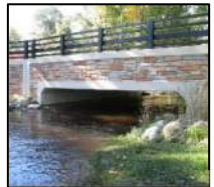
Figure 4: Three-sided box bridge
