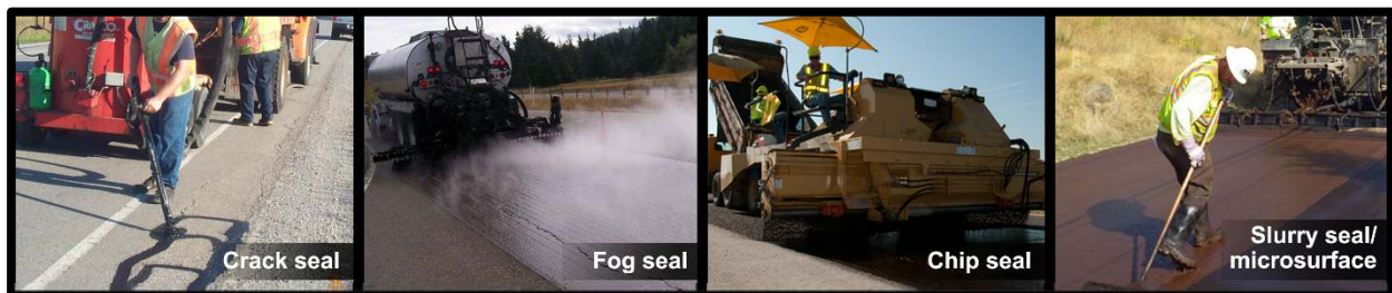
Figure 5: Examples of capital preventive maintenance treatments—(from left) crack seal, fog seal, chip seal, and slurry seal/microsurface.
