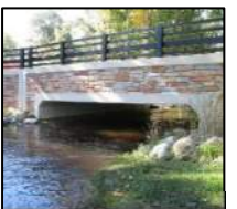
Figure 4: Three-sided box bridge
