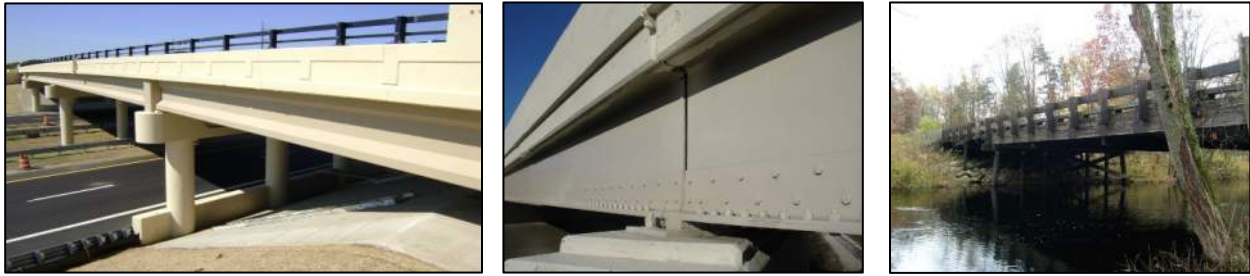
Figure 5: Examples of common bridge construction materials used in Michigan
